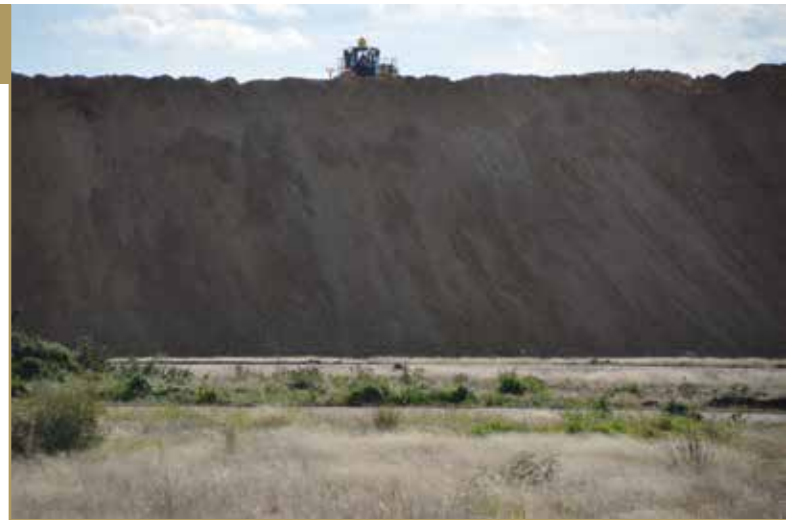
WRE 2 noise bund in place
